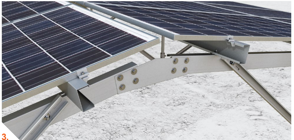
2. Detail of fastening panels to longitudinal profiles profily
